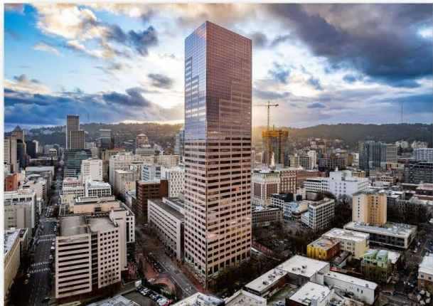
US Bancorp Tower
