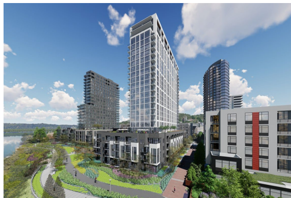
Willamette Tower — 23 story high-rise 343 units, 3,800 SF retail space.
